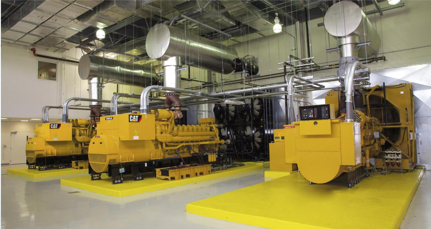
**The generator room houses two 5 Kv 3.0 Mw generators powered by 4423 HP diesel engines and one 2.25 Mw unit powered by a 3100 HP diesel engine.**
