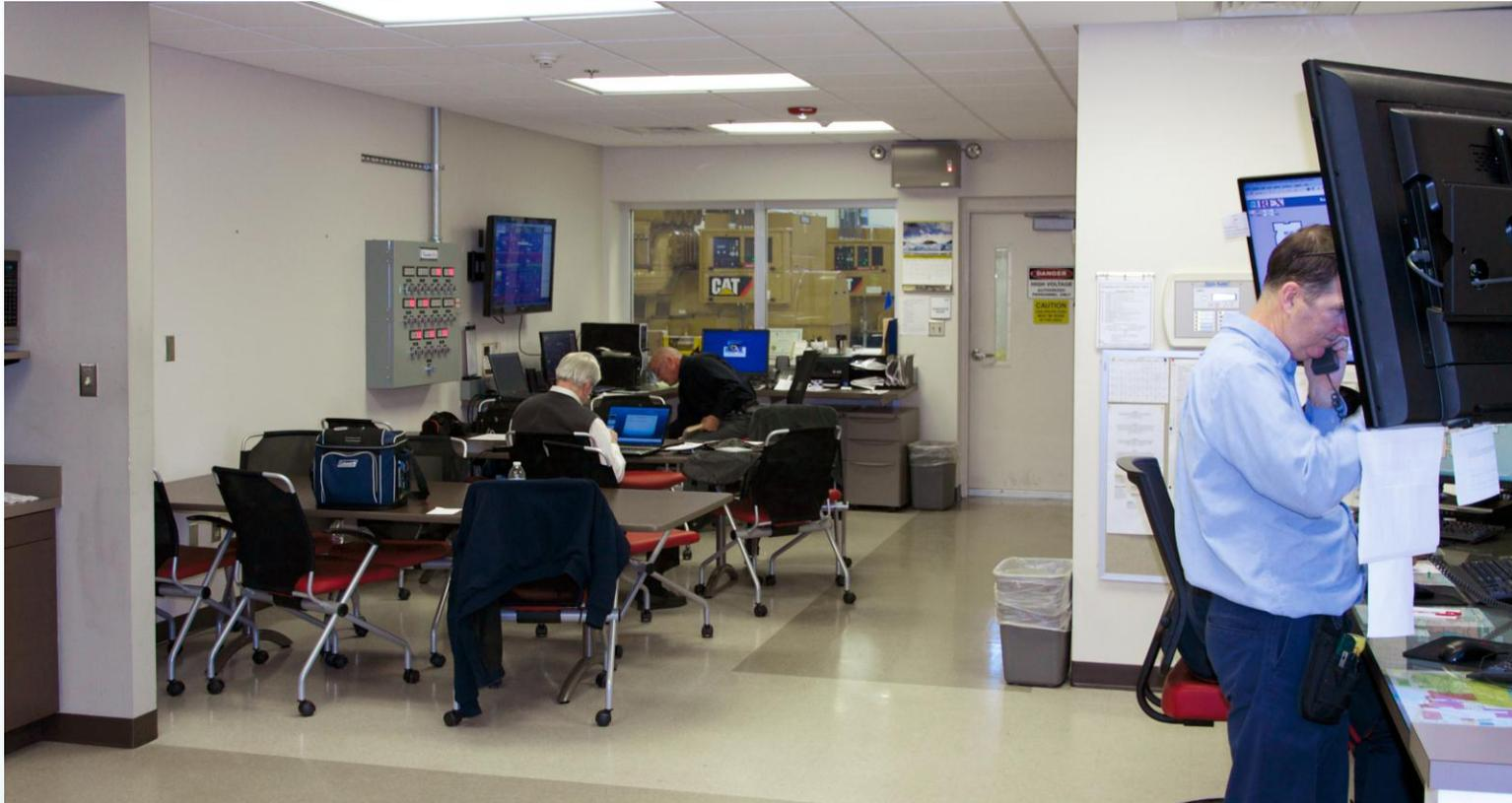
**The control room consists of a main control panel screen with the system 5 Kv one line diagram, multiple monitoring screens for engines, generators, switchgear, and data. The control panel also displays operating screens for controlling the system in either an automatic or manual mode.**
