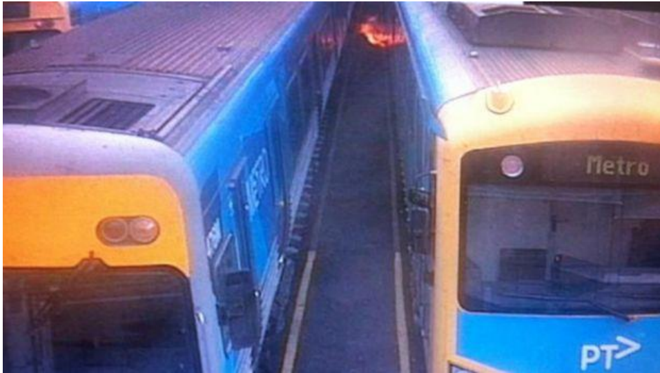
CCTV of Inverter Exploding [1]
